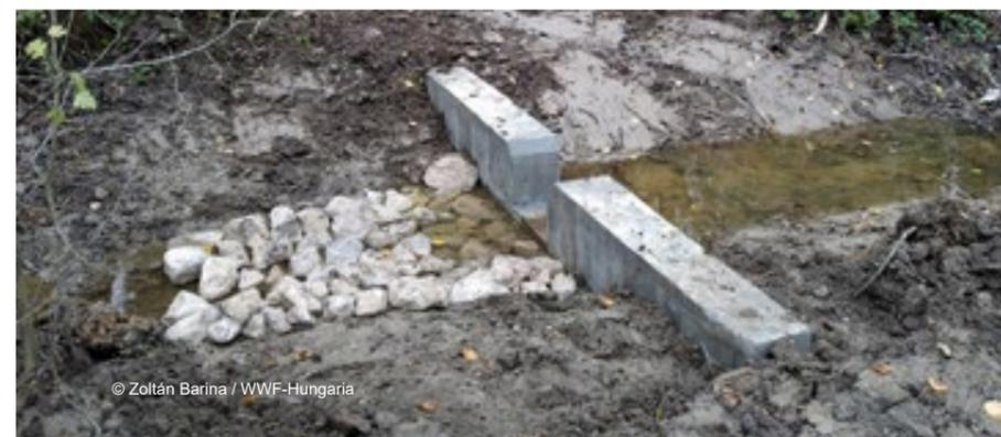
**SIX BOTTOM WEIRS WITH ADJUSTABLE SLUICES HAVE BEEN INSTALLED TO RAISE WATER LEVELS.**
